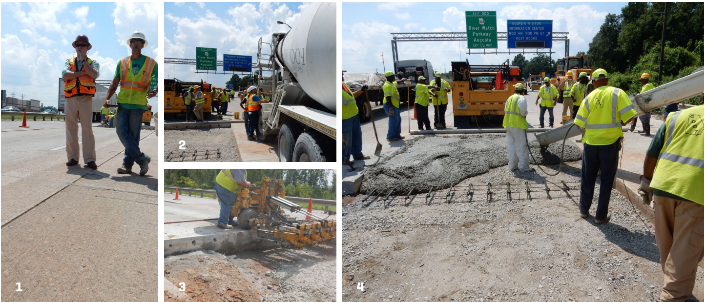
1, 2, 3, 4. EdenCrete® enhances concrete performance and does not affect the fresh concrete properties or its ability to be finished, which makes it extremely user-friendly to finishers on the job site.
